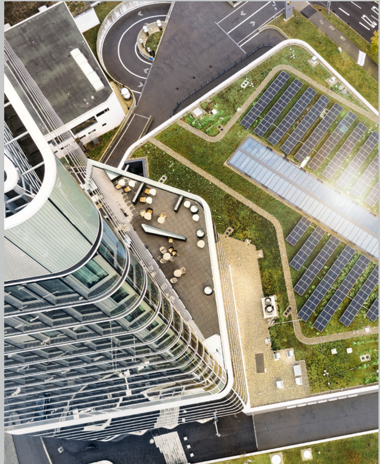
The Porsche Design Tower was planned with foresight—including a photovoltaic system on the roof of the Porsche Center Stuttgart
